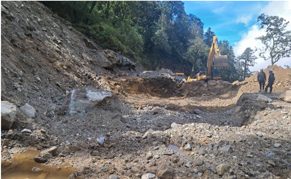
Figure 1: Excavation in desander area
