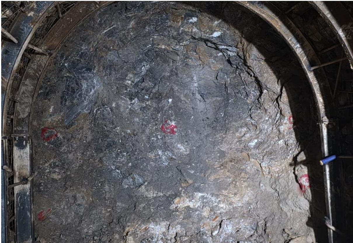
Figure 5: Inlet tunnel face at ch 0+109.50m
