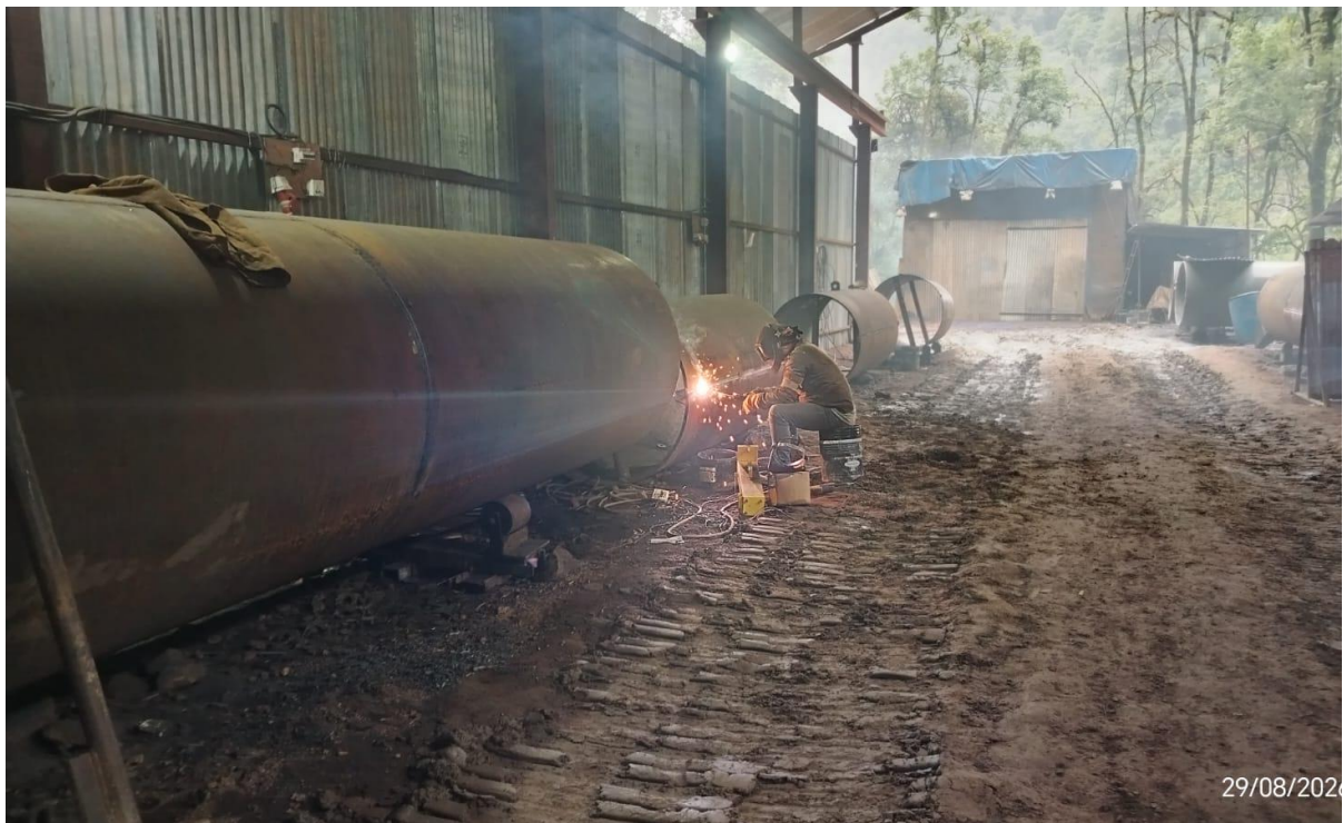
Figure 14: Welding in straight pipe in HM workshop
