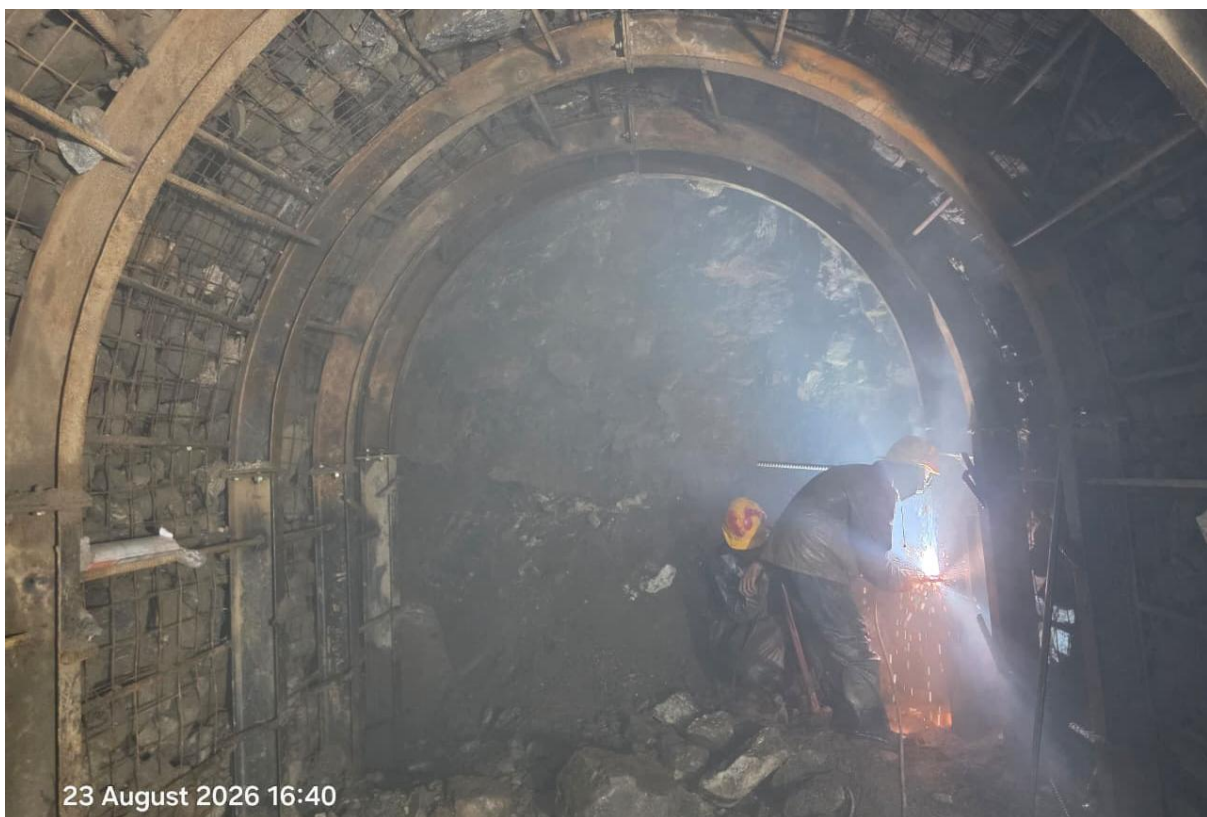
Figure 6: Rib installation work in Inlet tunnel
