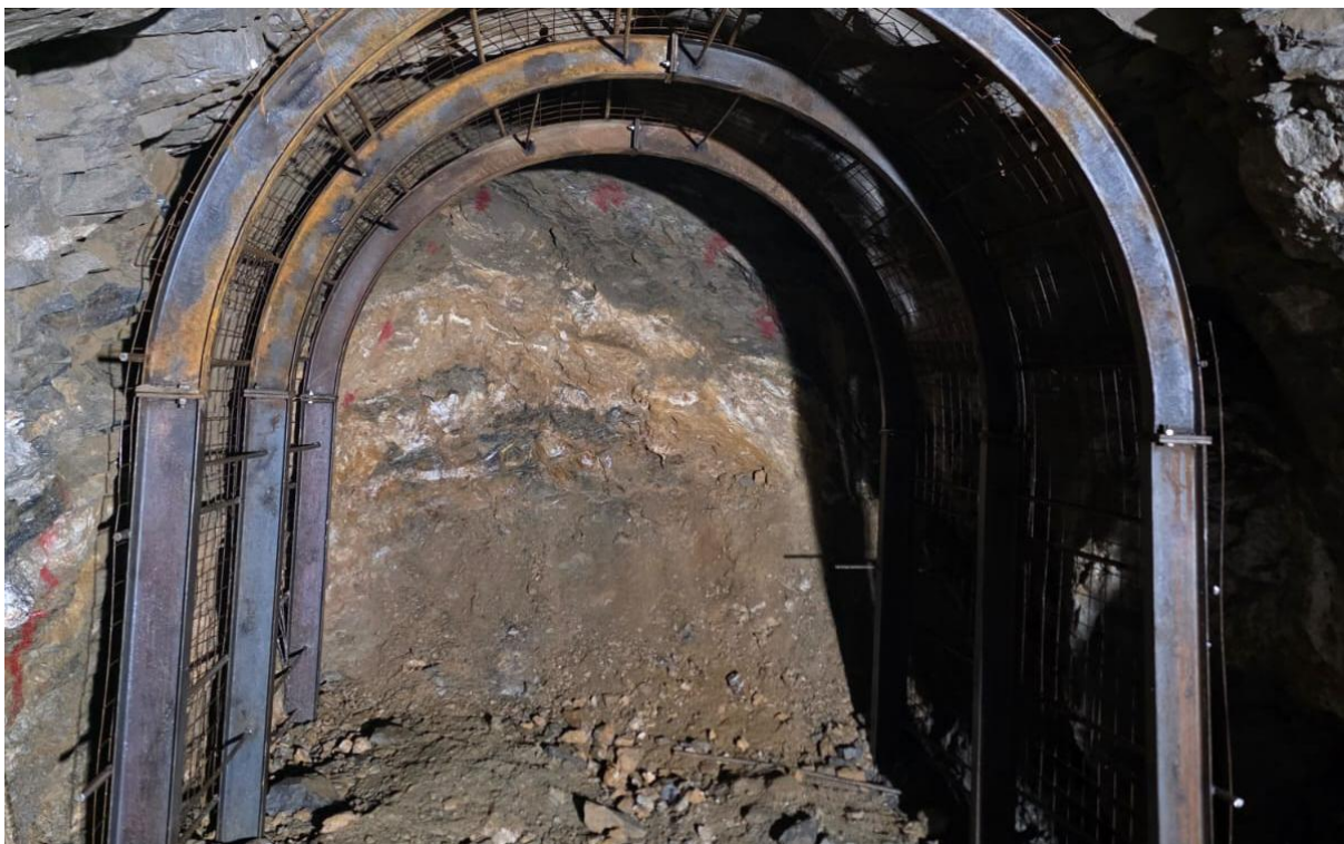
Figure 2: Concreting in wall of Undersluice u/s panel
