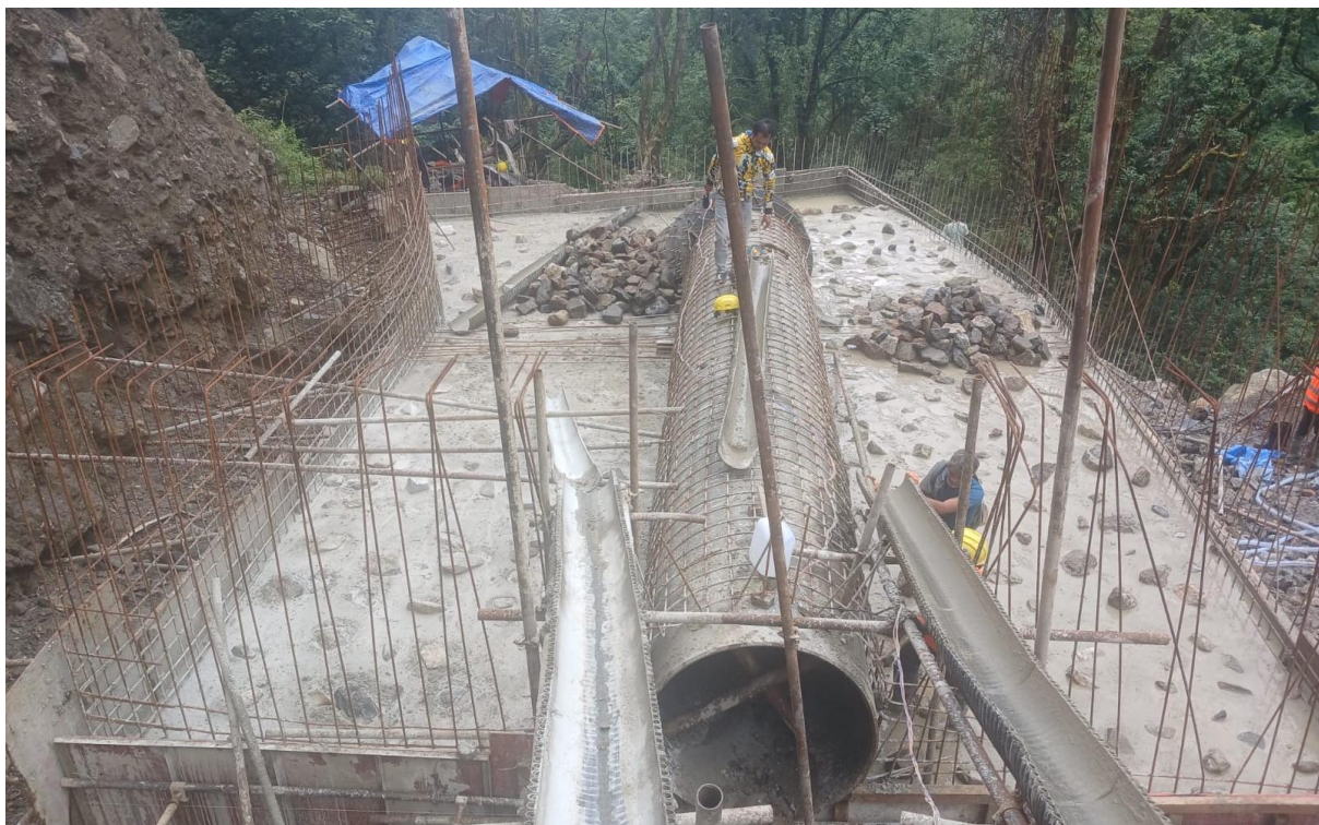
Figure 10: Plum concreting 2 nd lift in AB 12
