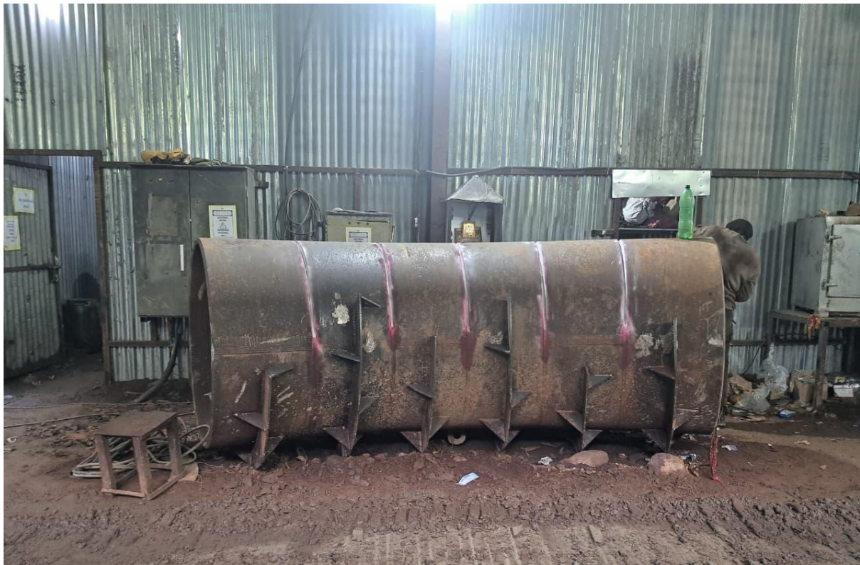
Figure 15: Welding in AB 11 bend in HM workshop
