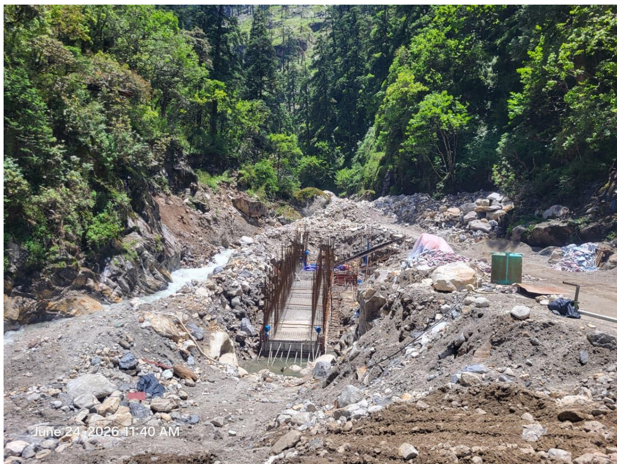
Construction of Nyadi Phidi Hydropower Project (21.4 MW)
