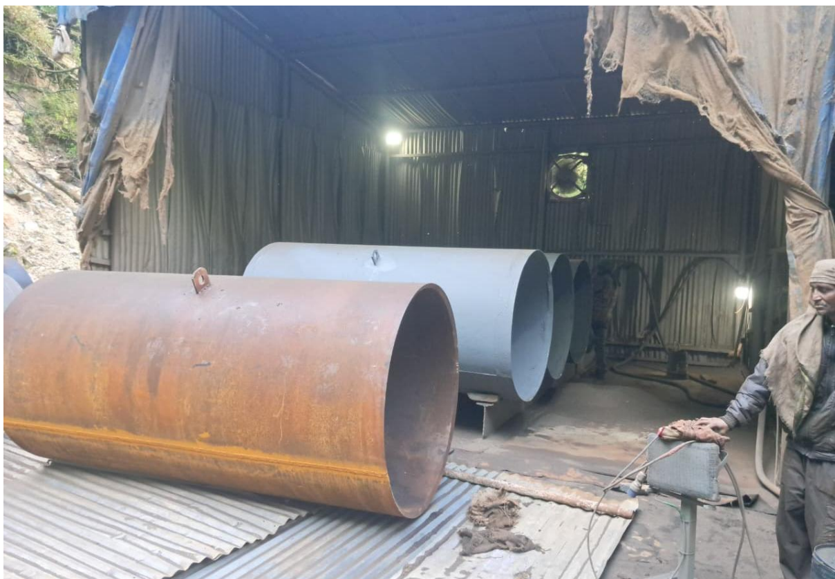
Figure 16: Primer coating after sand blasting in HM workshop
