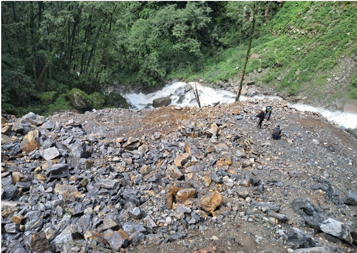
Figure 11: Survey work in powerhouse area
