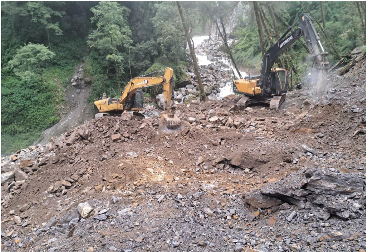
Figure 13: Powerhouse area excavation using breaker
