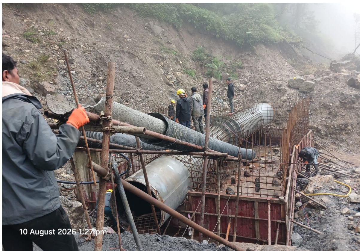
Figure 7: Rebar work and formwork in AB 9
