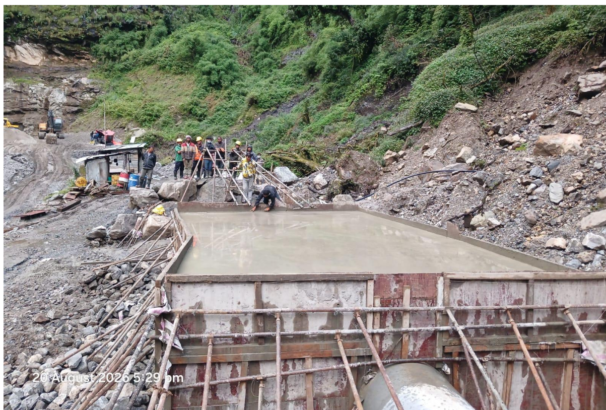
Figure 8: Plum concreting completed in AB 9
