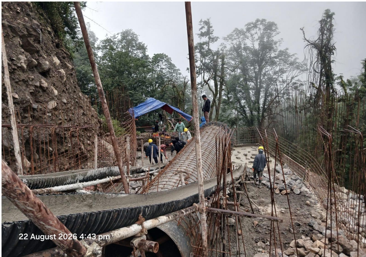
Figure 9: Plum concreting in AB 12
