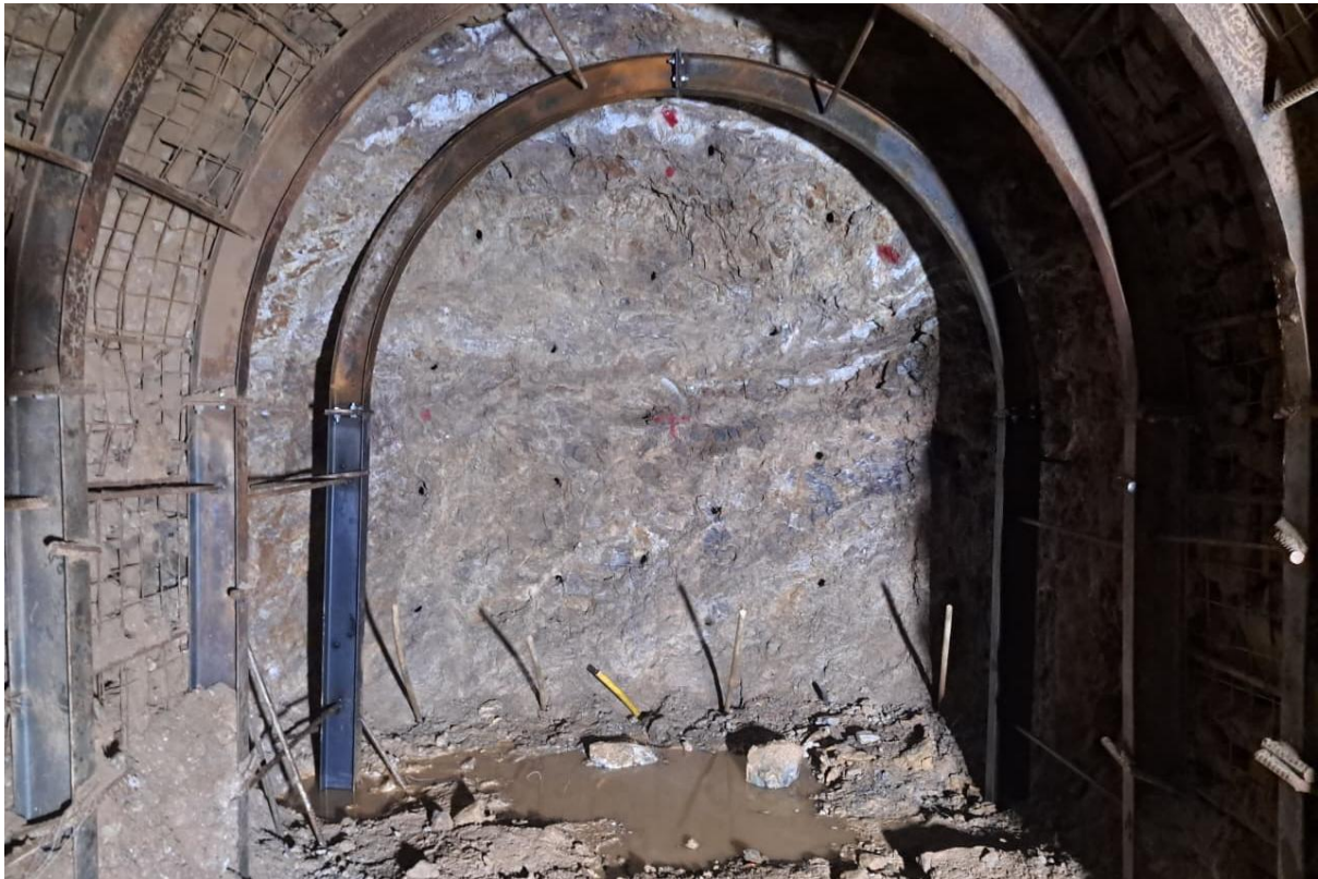
Figure 3: Excavation in Inlet tunnel at ch 0+104.25m
