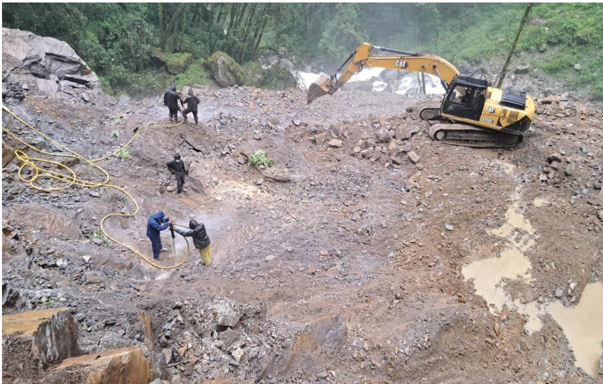
Figure 12: Drilling in powerhouse area
