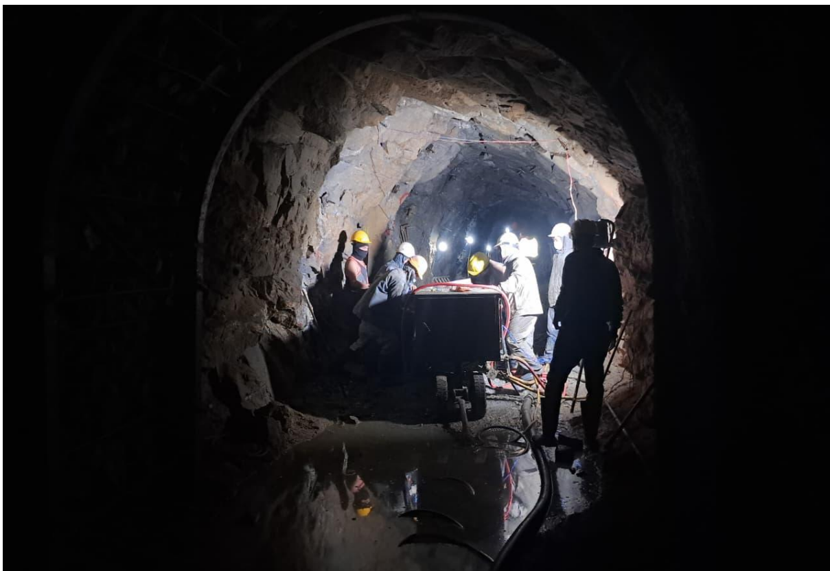
Figure 4: Preparation of shotcreting in Inlet tunnel
